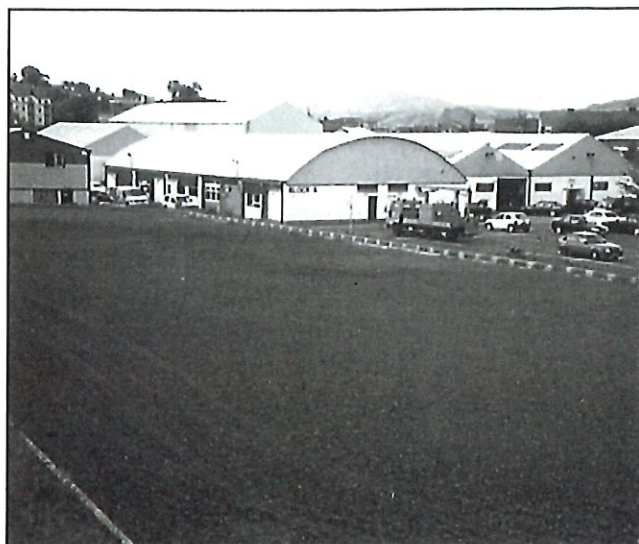
Site Preparations for a further large scale development at WIN Business Park which will be completed in 2002
