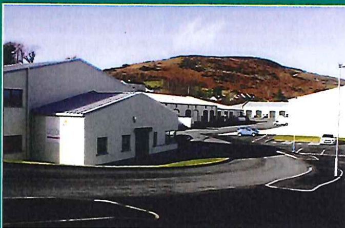
Flurrybridge Enterprise Centre
