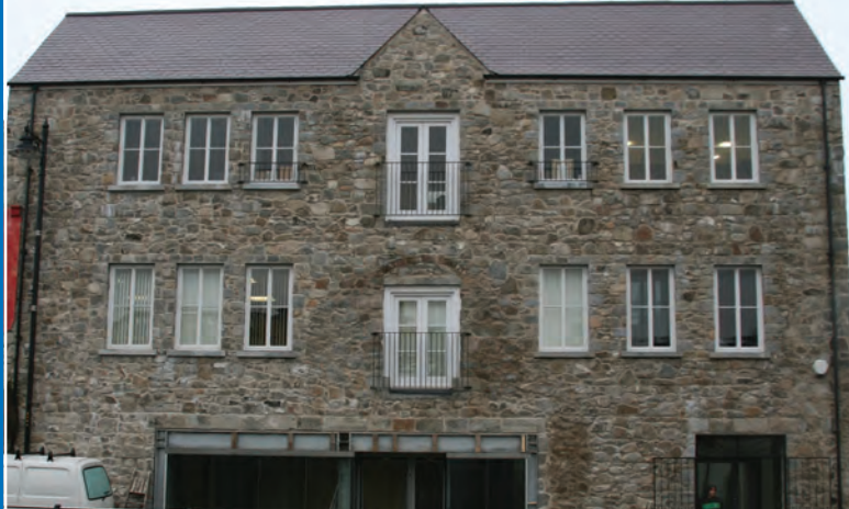
The First Derivatives headquarters building, Canal Quay, Newry.
