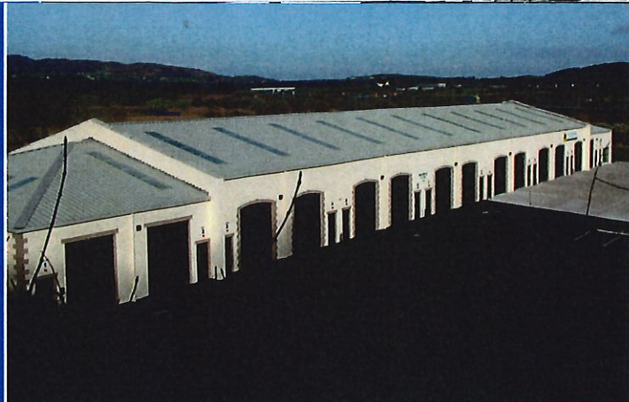
The new block which was completed at Flurrybridge
