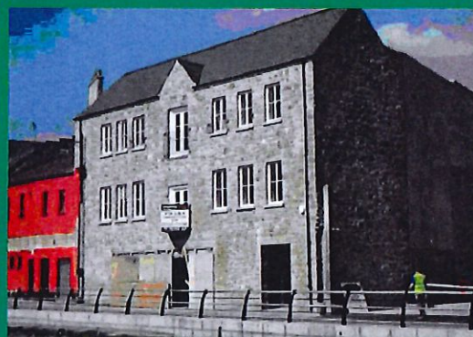
The refurbishment of 3 Canal Quay was completed during the year
