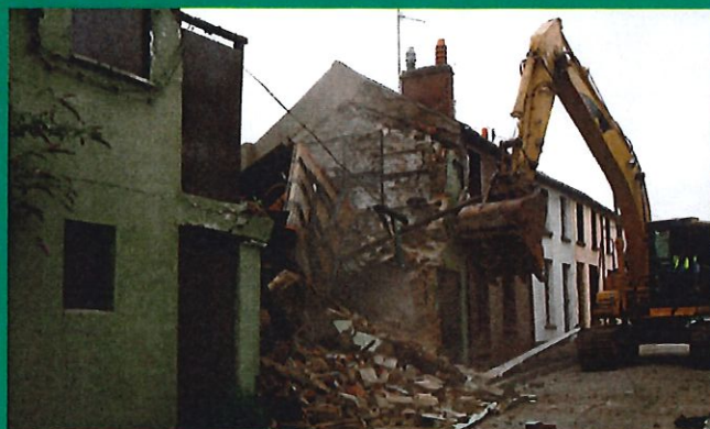
Housing redevelopment underway in lower Canal Street
